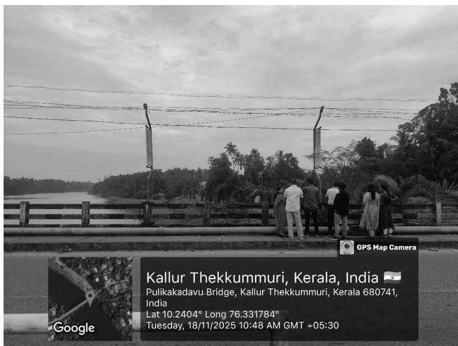
Joint inspection conducted at Pulikkakadavu bridge on 18.11.2025
