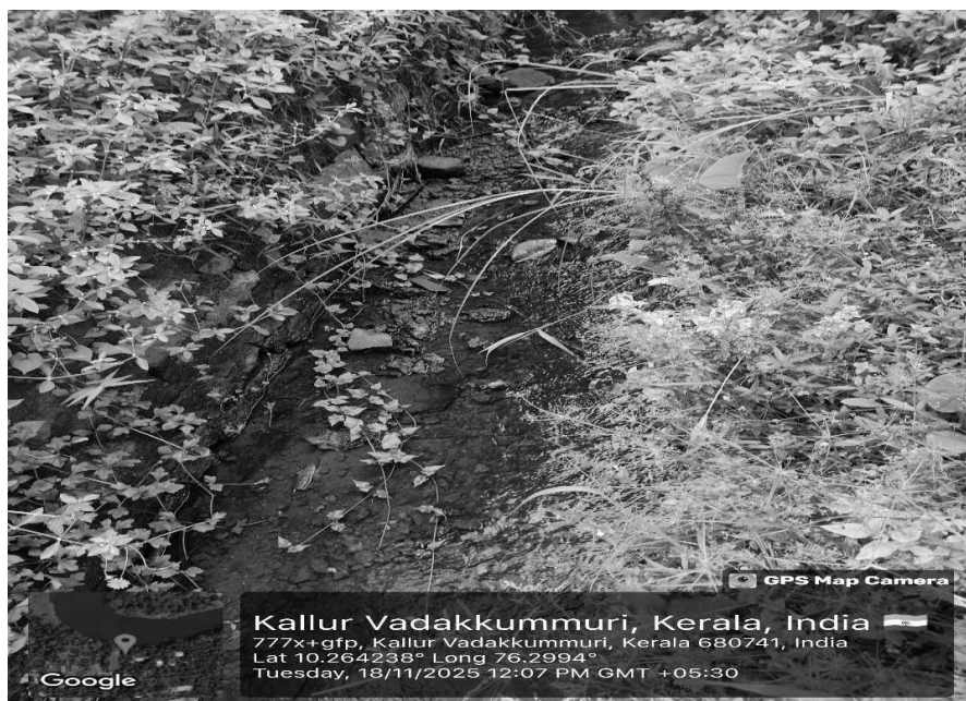
Drain located at Kallur Vadakkummuri during joint monitoring
